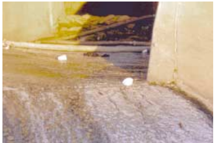
(Above) Runoff from the 8th Street drain. The grey substance coating the drain's ramp is bacteria feeding off of organic matter found in street runoff. A press conference was held at the site (below) to announce the joint project with local and state agencies.
